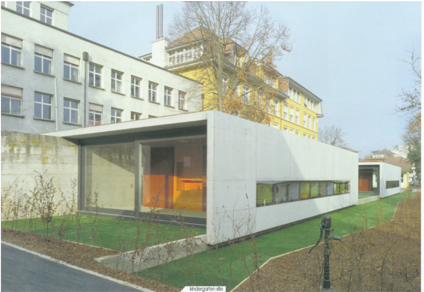
a platform in the ground, bordered by washed concrete forms the basis
